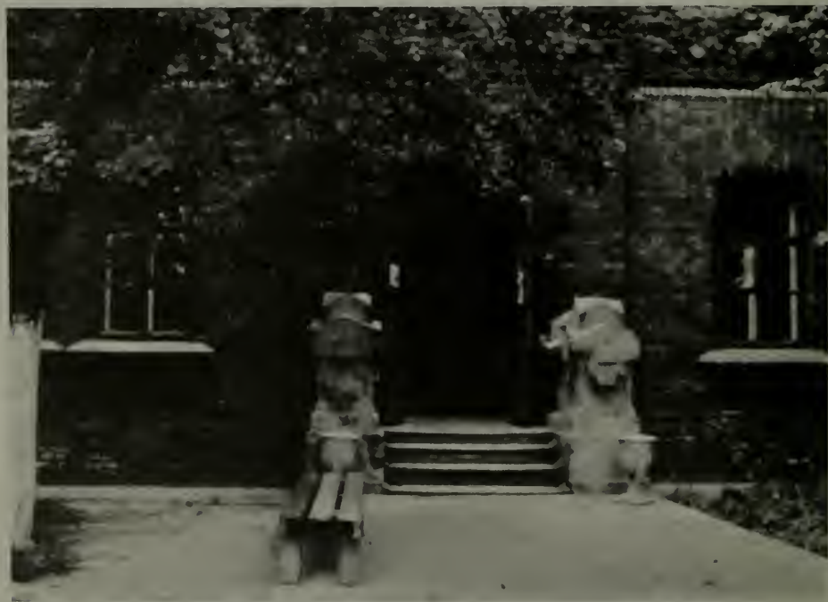
Entrance to one of the Kaschenko Hospital buildings.
